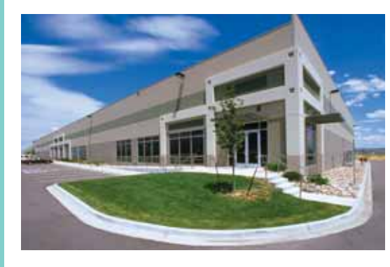
Compark Industrial Complex Englewood, Colo.
