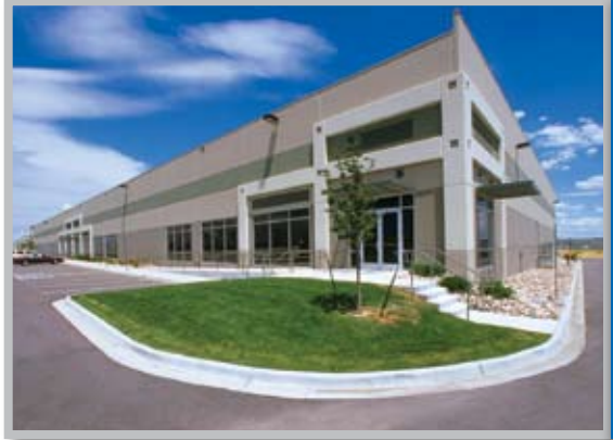
Compark Industrial Complex Englewood, Colo.
