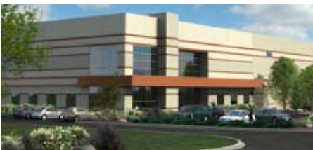
Opus Business Center at Rickenbacker – Building VI Groveport, Ohio
