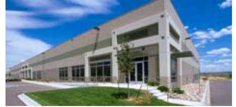
Compark Industrial Complex Englewood, Colo.
